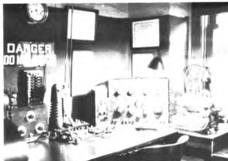
STATION - "WTK" CLEVELAND. It was installed in Room 1070 of the Cleveland Hotel. Picture taken in May 1925.
